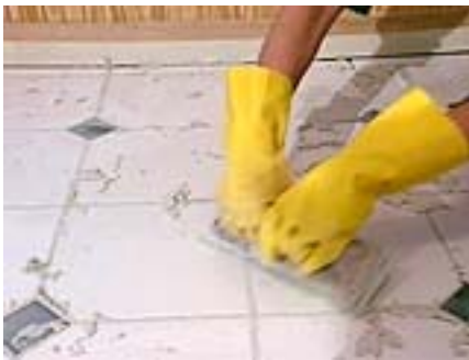
Working grout into grout joints.
