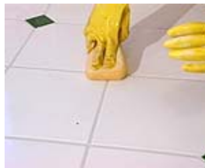
Clean grout off tile with clean damp sponge.
